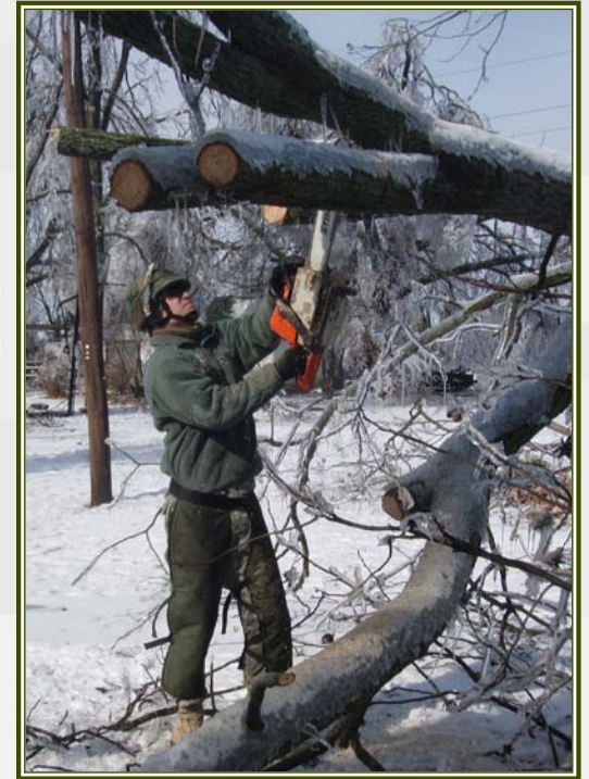
Patrick Phillips, of the 1138th Engineer Company, cuts away debris to clear a path following the January 2008 ice storm in Bertrand, MO.
