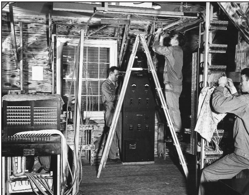
Switchboard maintenance at Camp Crowder, Missouri in 1943. U.S. Army Signal Corps photograph.
