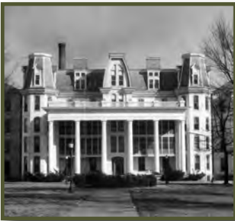
Fulton State Hospital Administration Building — Missouri State Archives
