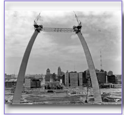
Construction of The Gateway Arch Missouri State Archives
