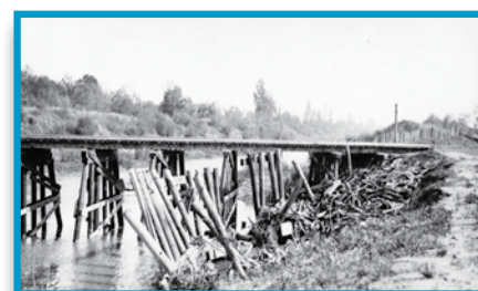
Trestle Construction in Southeast Missouri Missouri State Archives
