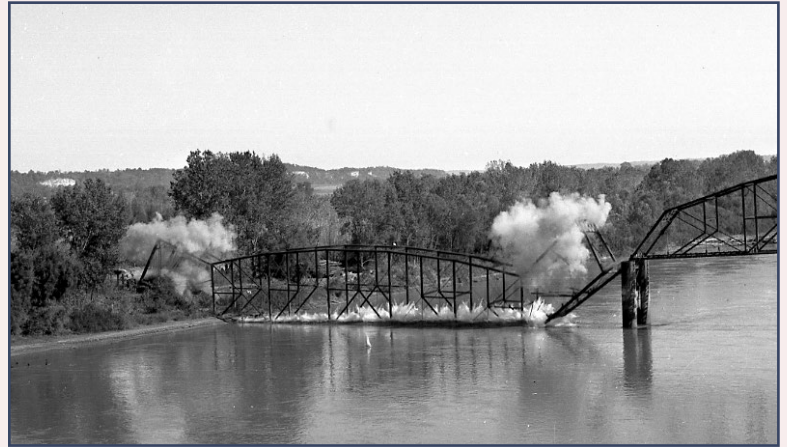
Demolition of the 1896 bridge, October 19, 1955.
