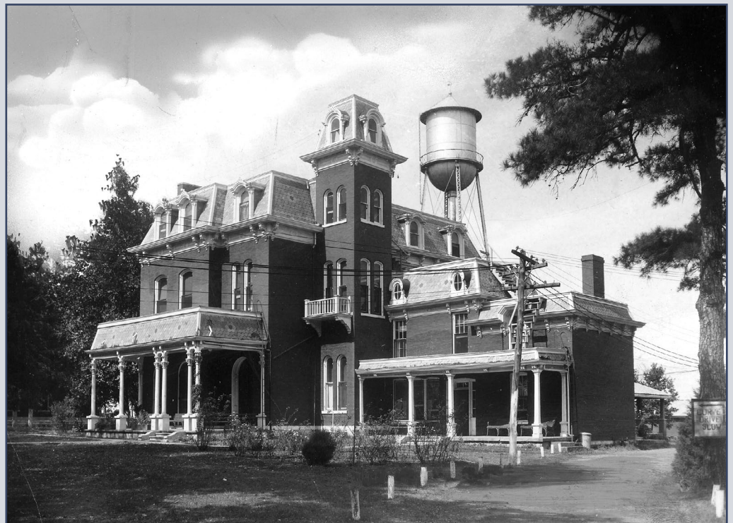
Below: William James originally built the Dunmoor Mansion (below) as a home in 1866. The mansion became the Federal Soldiers Home on October 25, 1896. Missouri State Archives.
