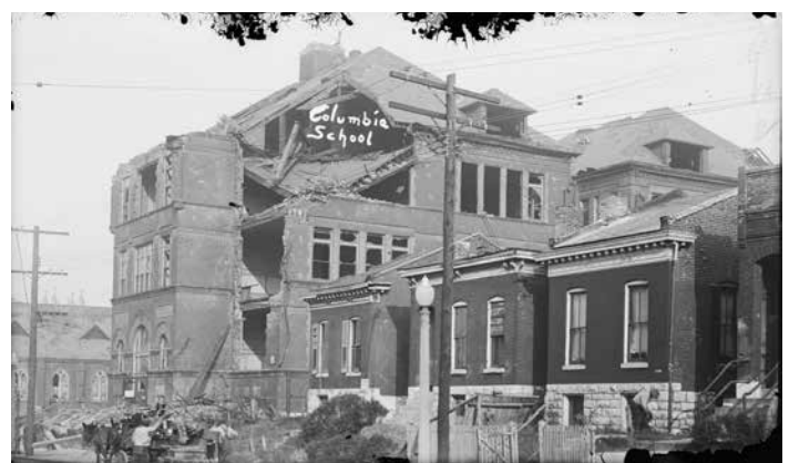
Glass plate photograph showing damage incurred by the Columbia School in St. Louis from a 1927 tornado. Fortunately, all 700 of the school's students survived. This and 32 other post-tornado images from the William A. Gearon Manuscript Collection are now available on the Missouri State Archives' Flickr page ( www.flickr.com/photos/missouristatearchives/ ).
