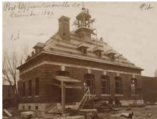
Above: Image of Kirksville Post Office under construction, 12/1904. Source: City of Kirksville Photograph Collection, Kirksville City Clerk and Missouri State Archives
