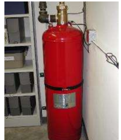
An example of the storage canister used in gas a fire suppression system
