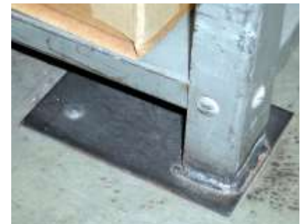
A shelving unit bolted to the floor for in case of earthquake
